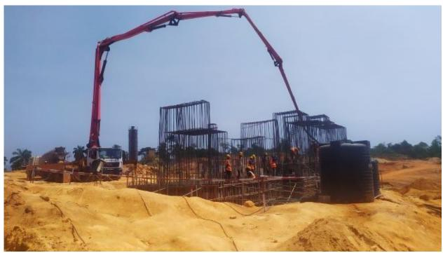
Figure 2: Casting of Ball Mill Foundation
